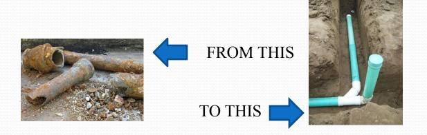
846 Feet OF 4" and 6" cast iron or clay sewer laterals replaced with PVC within the road right of way
